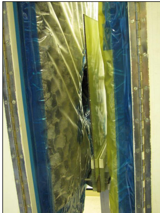
Figure 3. E glass panel placed in test assembly.
